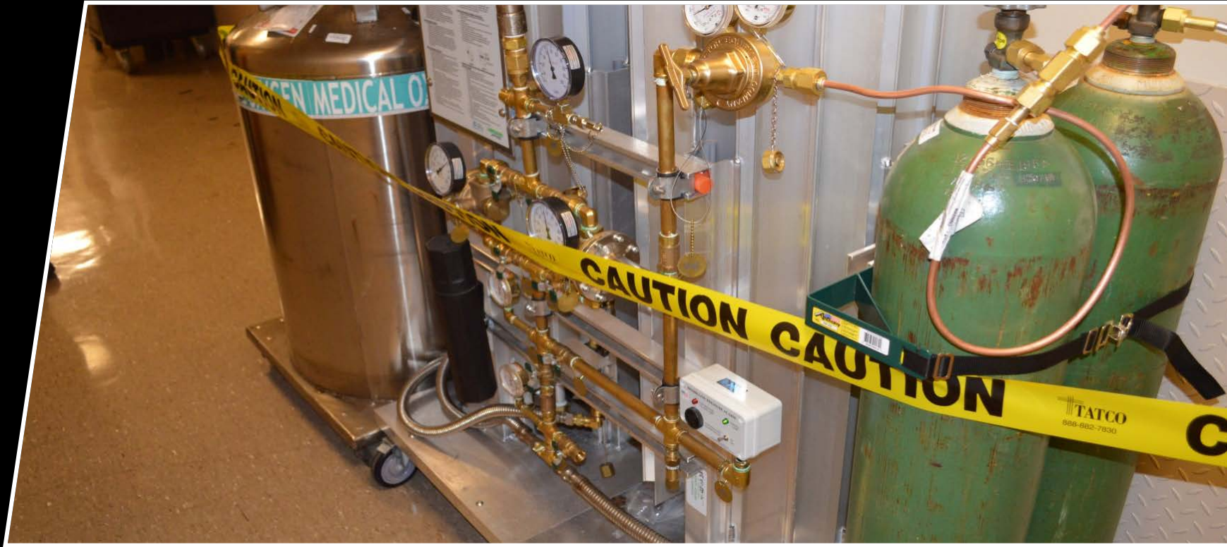
Emergency Oxygen Manifold in Use
