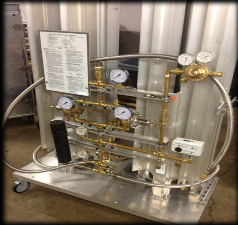
Emergency Oxygen Supply Manifolds
